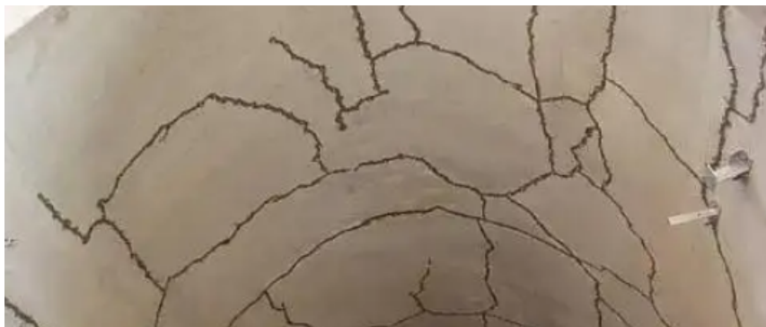
Figure 2. Secondary lining cracking in Jinfeng Tunnel
